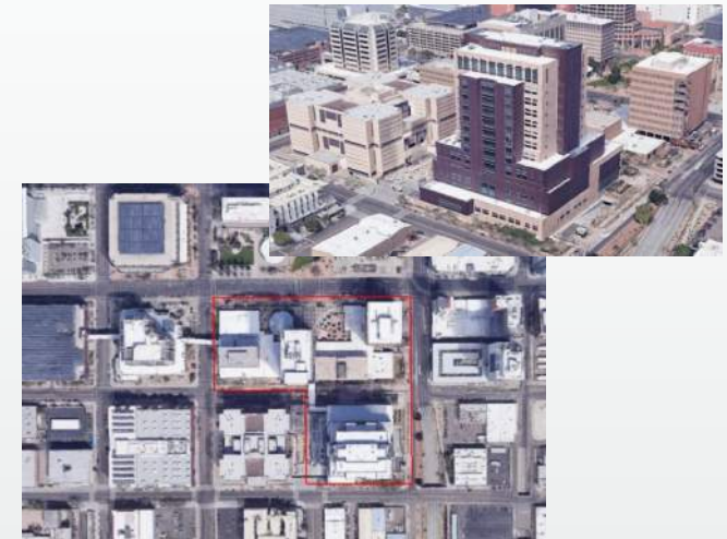
Maricopa County Courts Complex Phoenix, AZ 9.00 acres
